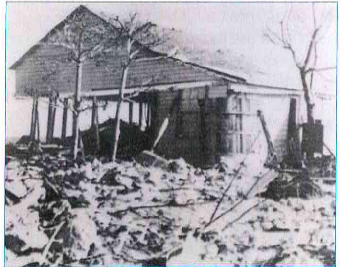
A house on Cayman Brac after the 1932 hurricane
